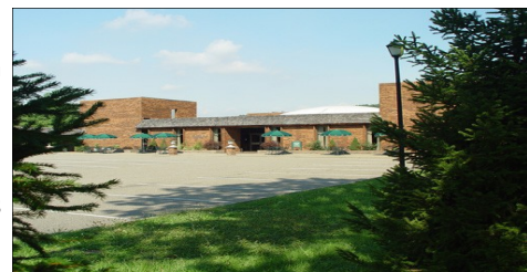
Mountainside Conference Center
